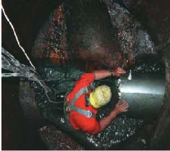
Sleeve installation in sewer. Transducers are pre-mounted on sleeve Model 7510 Multiple-Path Compound Transit-Time Flowmeter
